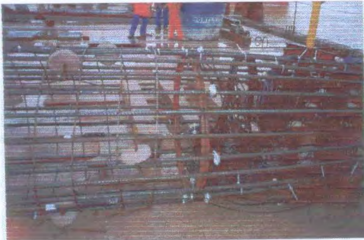
Photograph 2 – Sister Bars fixed inside cage
