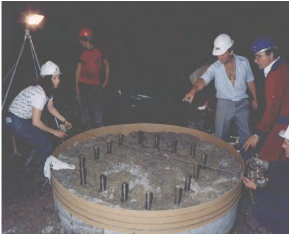
Figure 1 – Load cell fitted on pile top
