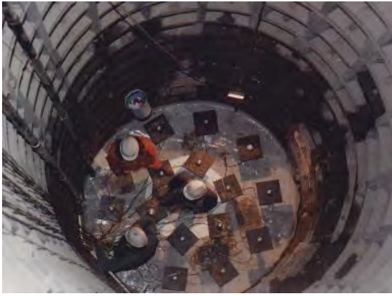
Figure 7 – Shaft load cell
