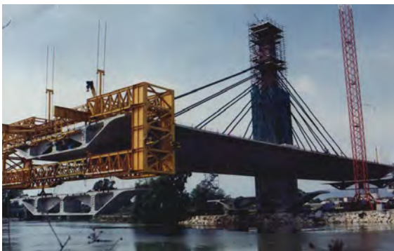
Figure 8 – General view of the Garigliano Road Bridge
