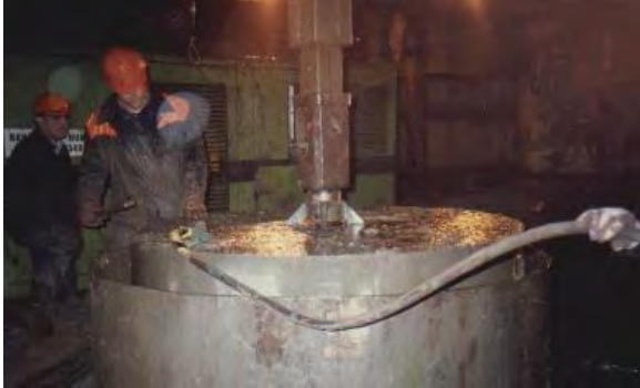
Figure 5 – Base load cell cast in concrete
